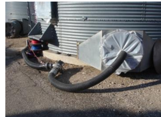
Sealed vent to bin aerating system
